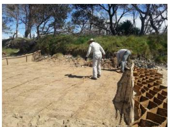
A set of 8—10 parallel fences was installed at Sandy Beach with widths of hessian attached to timber posts and jute material pinned onto the sand in between fences (on the left) and honeycomb patterned thicker jute as an alternative (on the right).
